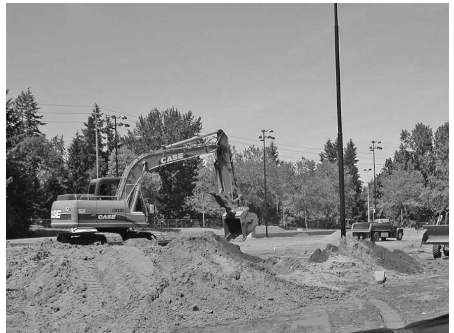
*Robinswood Park's fields are regraded in preparation for installation of synthetic turf.*
