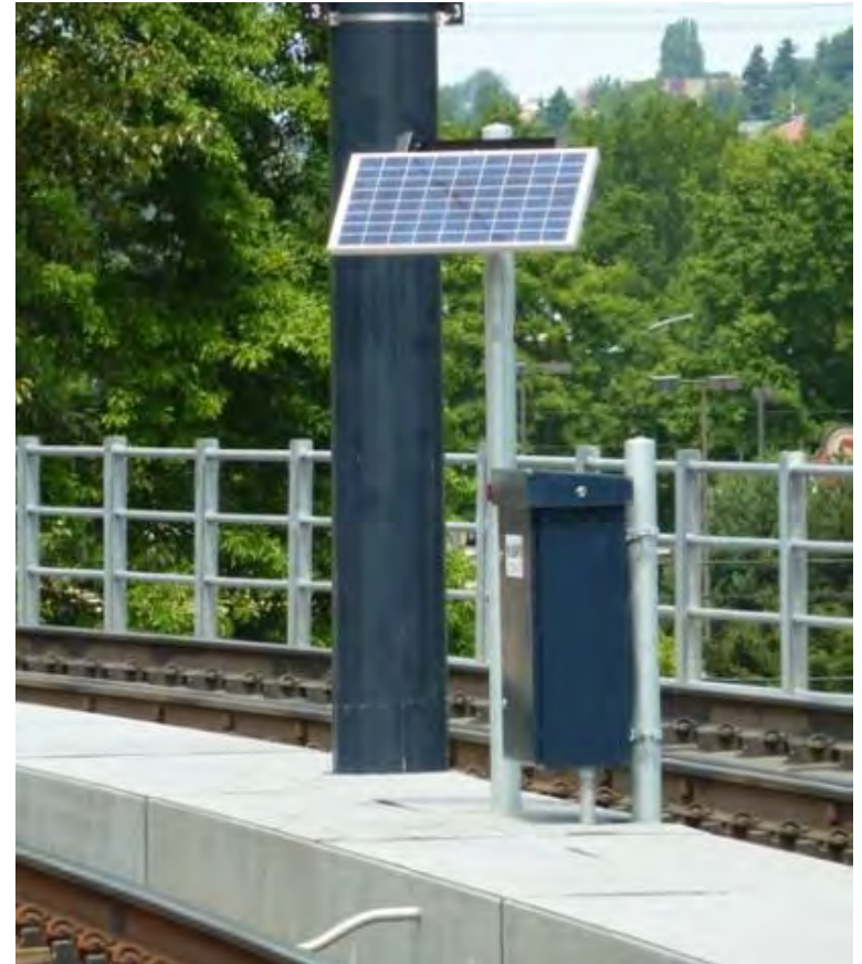
Solar Rail Lubricator
