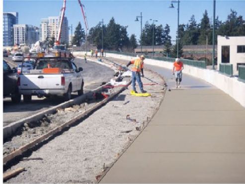
Wide Path on Main Street Bridge
