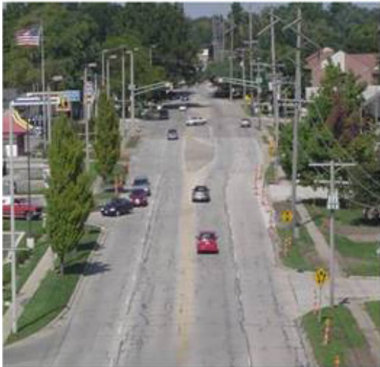
BEFORE: Four lanes without center turn lanes
