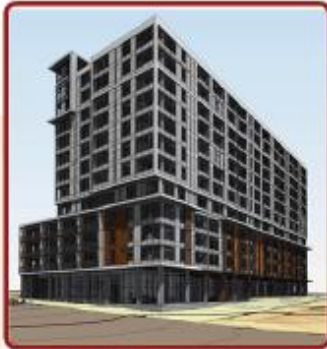
5 Alley 111 11011 NE 9th Street
