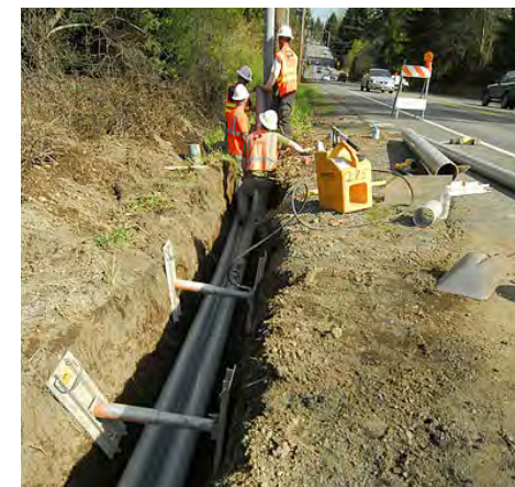
Underground distribution cable replacement
