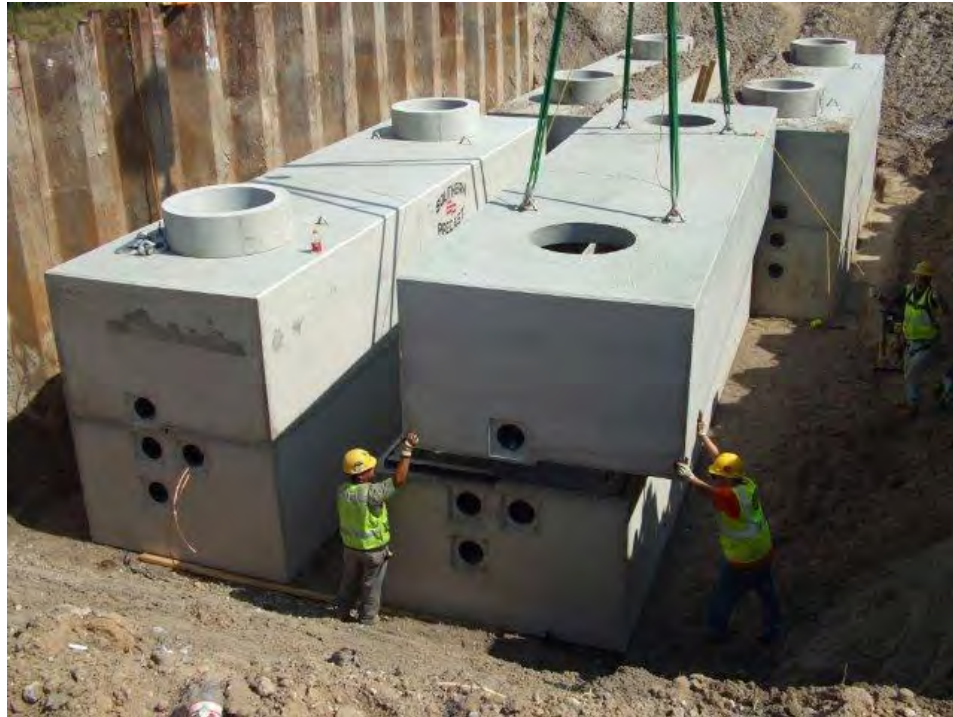
Splicing vault installation (Source: POWER Engineers)
