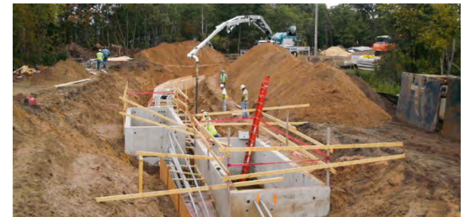
Transmission duct bank and vault placement (Source: POWER Engineers)
