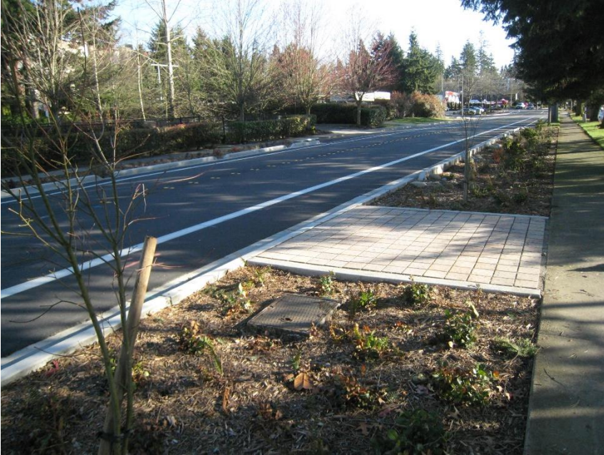
Redmond Overlake Village LID Roadway Retrofit
