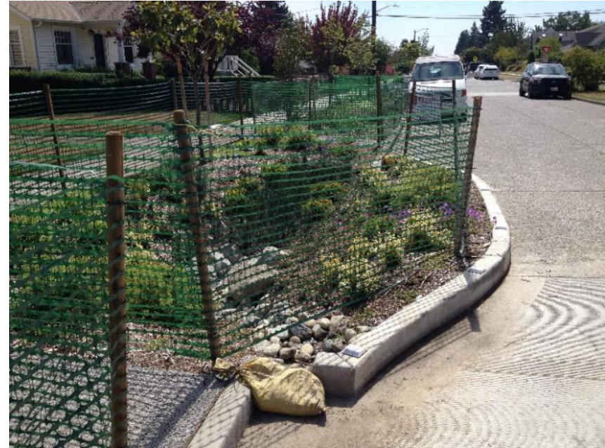
Sand bags prevent silt-laden flow from entering the bioretention facility. Green construction fencing prevents compaction due to foot traffic.
